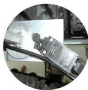
梯级（踏板）下陷保护装置 Step (tread) sunk protection device
